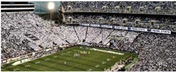
Rendering shows how electronic signs will light up the end zones of Beaver Stadium this fall.
